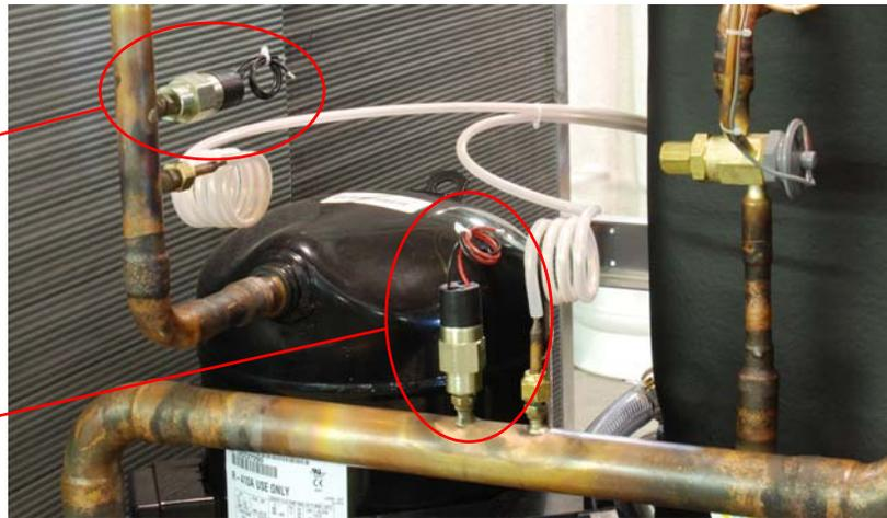
Typical placement of non-adjustable "fixed" pressure switches.
