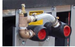
Typical optional automatic low flow bypass valve.
